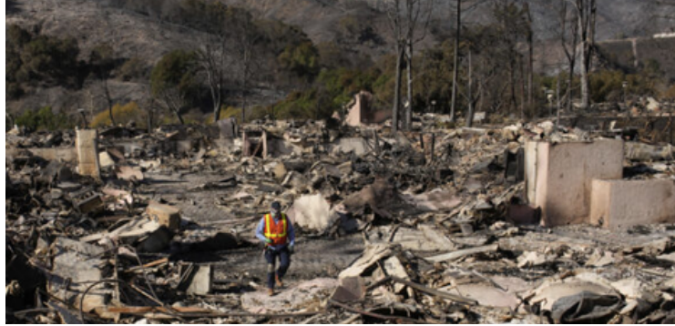
A worker surveys the damage from the Palisades Fire in the Pacific Palisades neighborhood of Los Angeles on Jan. 13, 2025. (AP Photo/John Locher, File)
